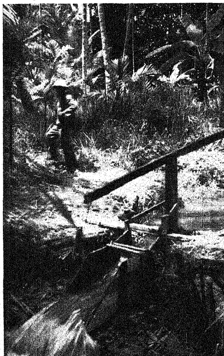
Figure 50. A wooden tilting bucket, counterweighted, for automatic flushing of small streams. Bucket in lowered position, discharging flush water
